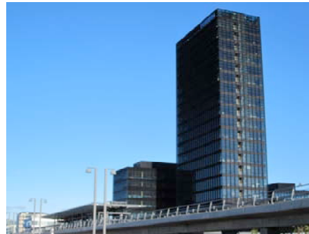
4| Ferring International Centre and Metro station Ørestad, ref. parts two, three
