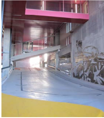
7 | View of the parking space in the residence Bjerget, part two
