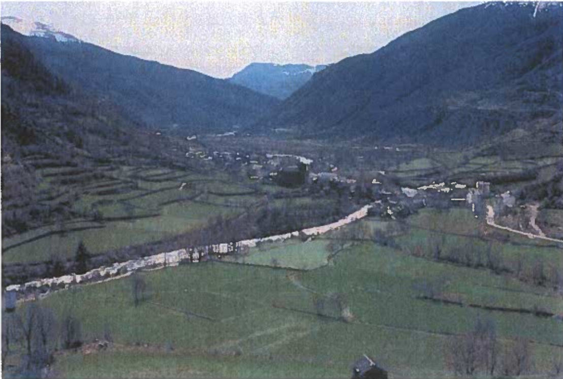
The Cohesion Fund also participates in achieving the objectives set out in the context of the Community's environmental and sustainable development policy. To tackle soil erosion, a levee is built in Spain, and a reforestation project is undertaken in the Ebro region.
