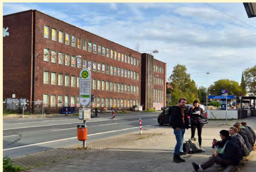
Site visit to a former steelworks production site in Bochum
