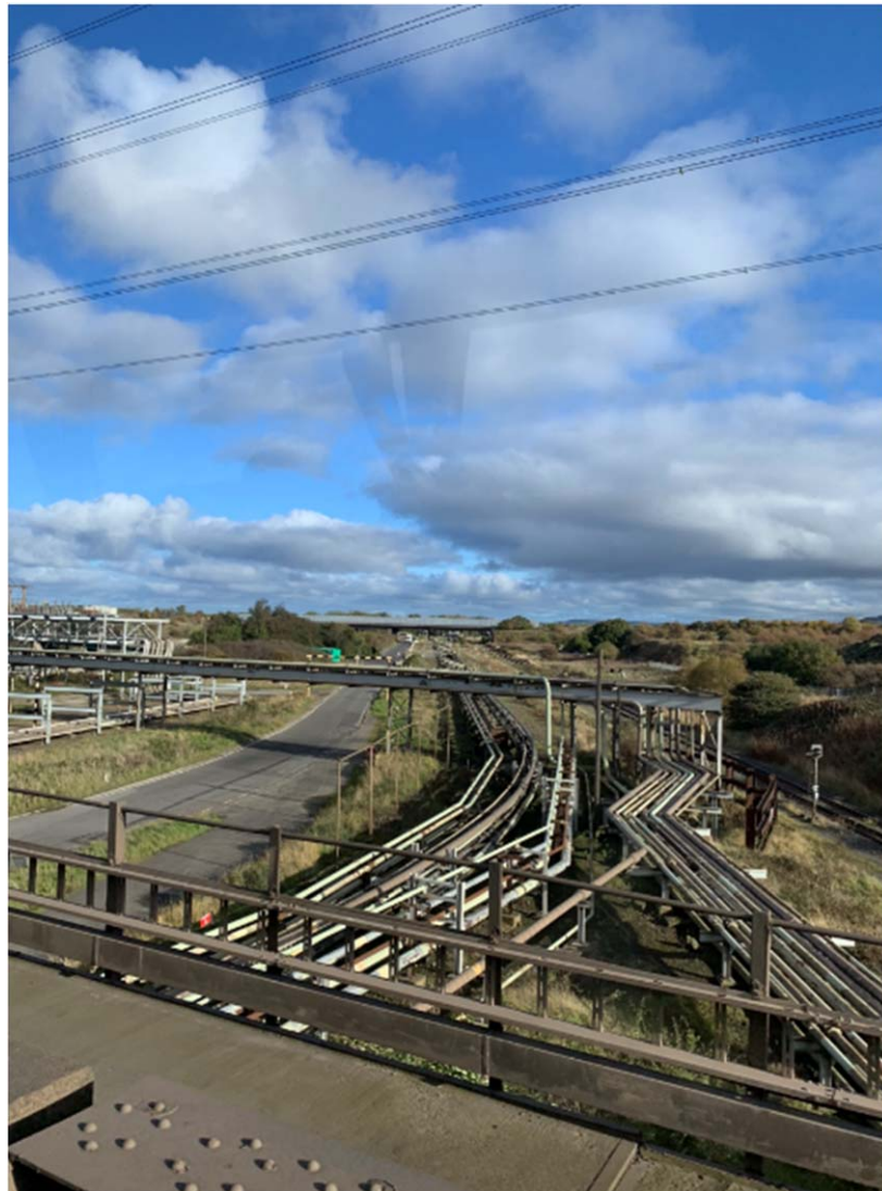
Figure B2. Vintage Pipelines in Teesworks.
