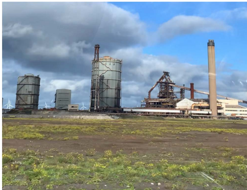
Figure B1. BOC industrial site, Teesworks complex.
