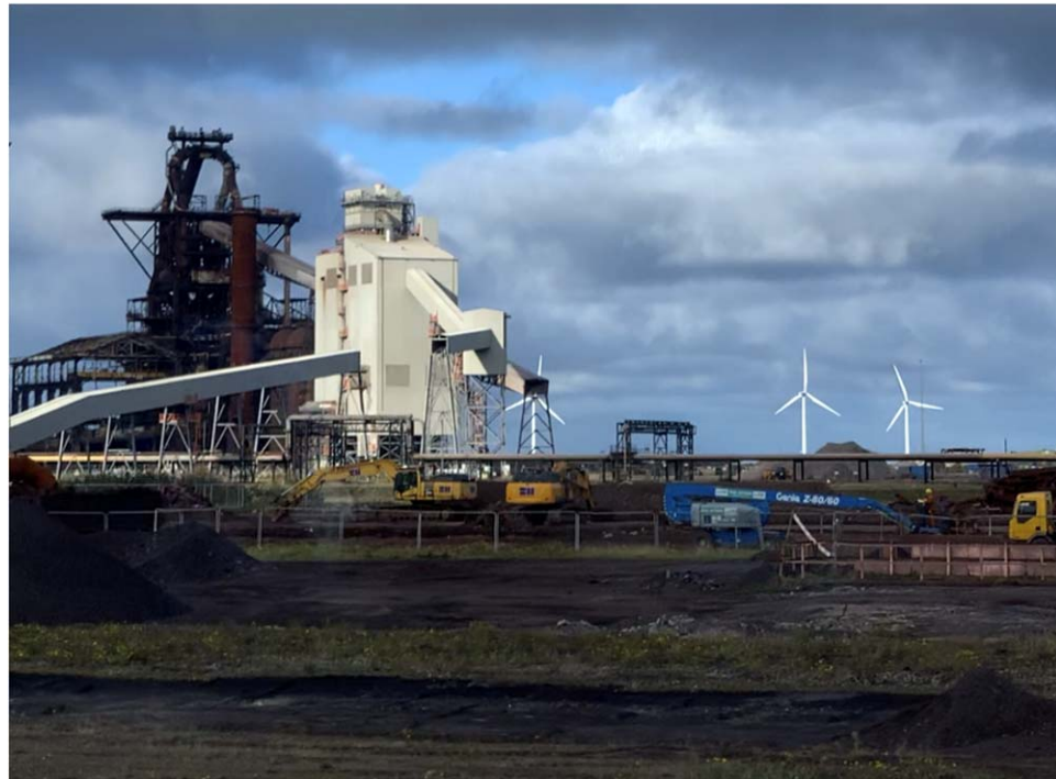
Figure B3. View of old industrial plants with wind energy in the background.
