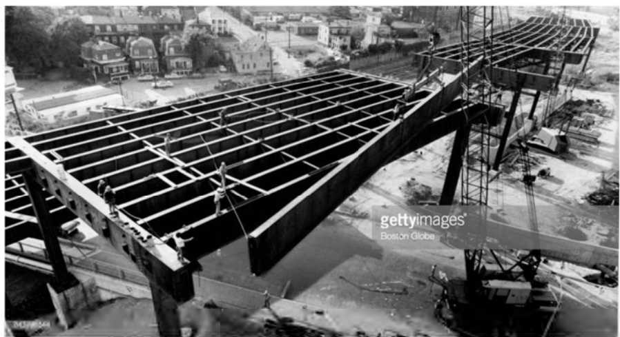
Fig. 4 - The construction of the Interstate 93. June 13, 1971, Photo by Ellis Herwig, The Boston Globe via Getty Images
