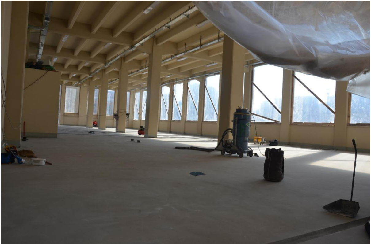
Figure 2 Via Cumiana structure. Source: site visit on February 13, 2020)
