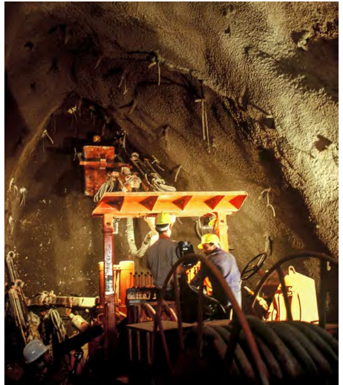
Starting in 1994 the Cohesion Fund provided financial aid to Member States with a per capita GDP of less than 90% of the EU average, i.e. Ireland, Greece, Spain and Portugal. In Spain this funding was notably used to build a new ring road around Madrid.
